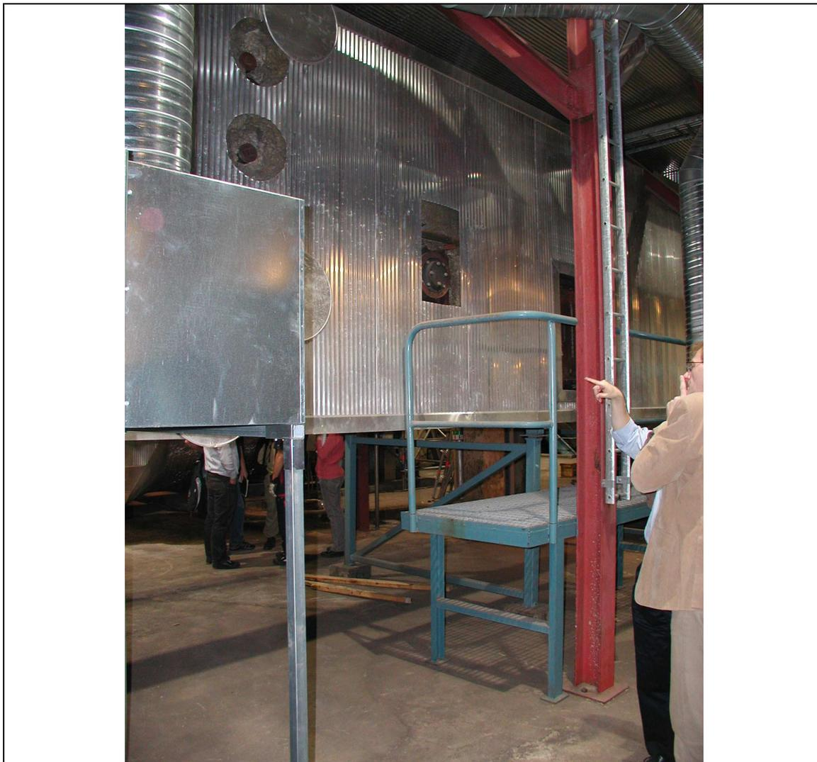
*Figure 2. A photograph showing the location of sampling points in the flue gas duct. The flow in the duct is from the right to the left and the ESP is to the left outside of the picture. The sampling points are from the left: the ordinary sampling cross-section with four ports in a vertical line, the blind flange where port A was opened and partly hidden behind the pillar, the man-hole where a port for the REMPI-TOF MS was opened.*
