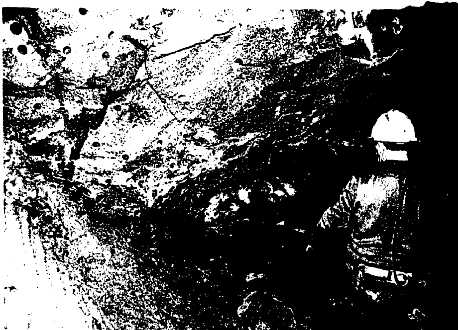
FIGURE 10: Photograph showing the rock splitters in use.
