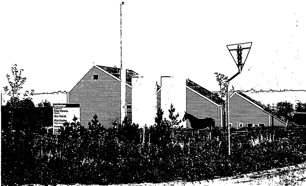
In Ærøskøbing the strawfired boiler covers 80% of the heating demand.
