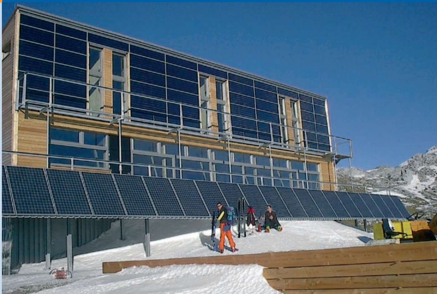
Fig. 3 - Schiestl-Haus: First Alpine Passive House, 2 156 meters high 7,5 kW PV (photo Fa. ATB Becker).
