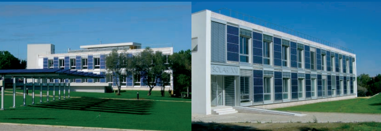
Fig. 1 - INETI installation: 12 kWp BIPV at INETI's Solar XXI Building (photo courtesy of INETI).
