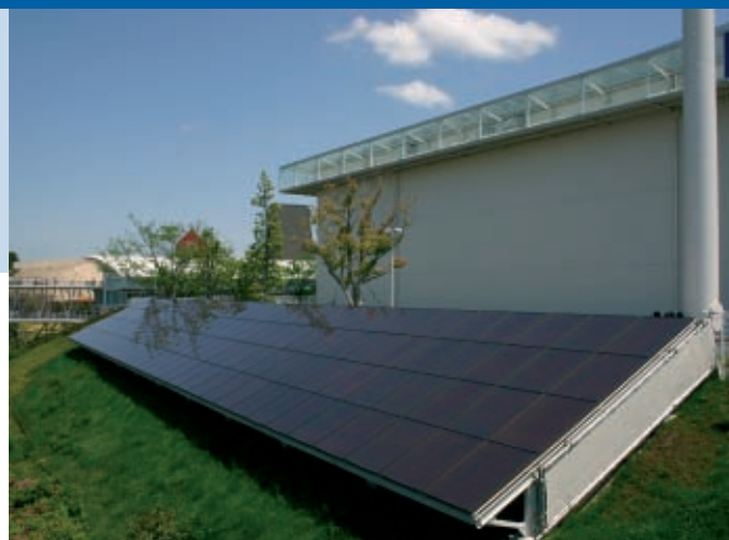
Fig. 3 - PV system installed on the slope, 100 kW, Aichi EXPO.
