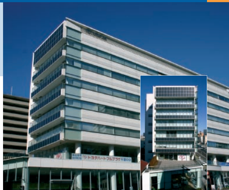
Fig. 6 - PV system at Chiba Toyota headquarters building, 10 kW, Chiba City, Chiba Prefecture.
