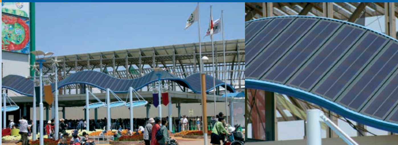
Fig. 2 - PV system using flexible type PV modules, 10 kW, Aichi EXPO.
