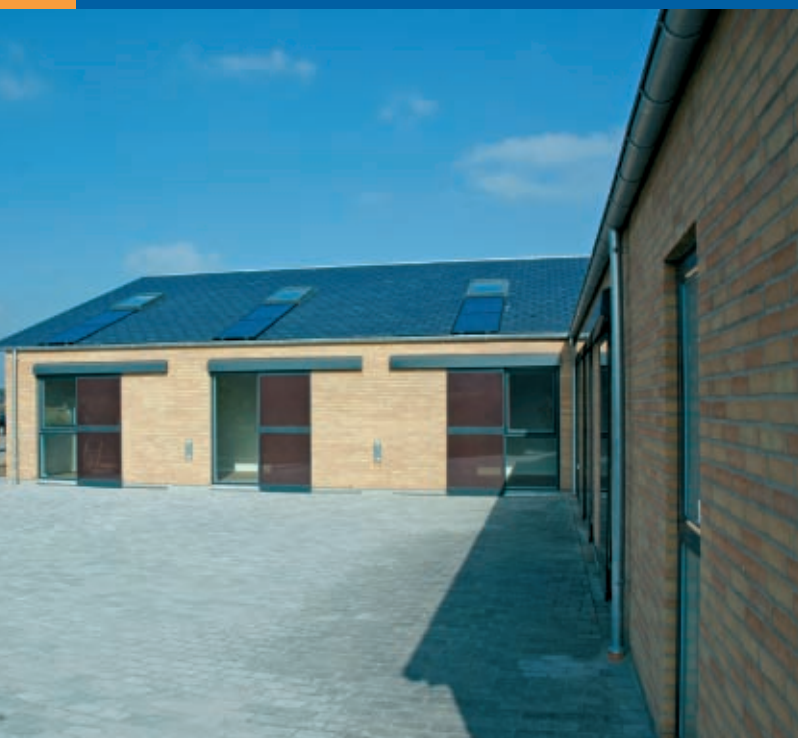
Fig. 2 - Solar cells integrated in the roof and transparent solar shutters.
