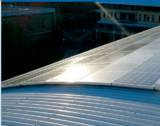
Fig. 2 - 42 kW grid connected PV array at University of NSW (photo BP Solar Australia).
