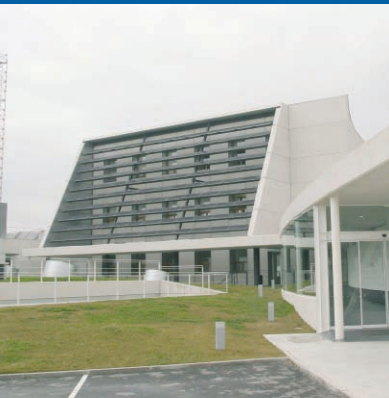
Fig. 1 - PV integration on façades at the CENER building.
