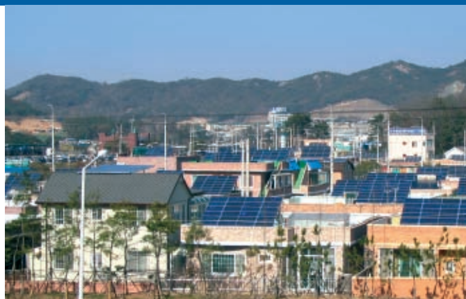
Fig. 1 - PV powered Green Village in Gwangju Metropolitan City under the 100 000 Rooftop Programme. Total 96,9 kW grid-connected PV systems are installed on the roof of 46 residential homes.
