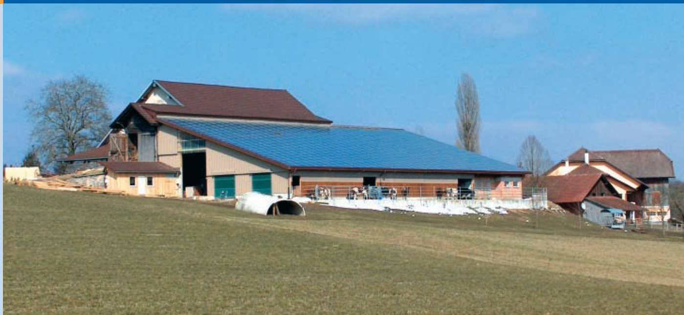
Fig. 2 - 110 kWp roof integration on a farmhouse with Solrif® frames (PV design: Solstis, photo NET).
