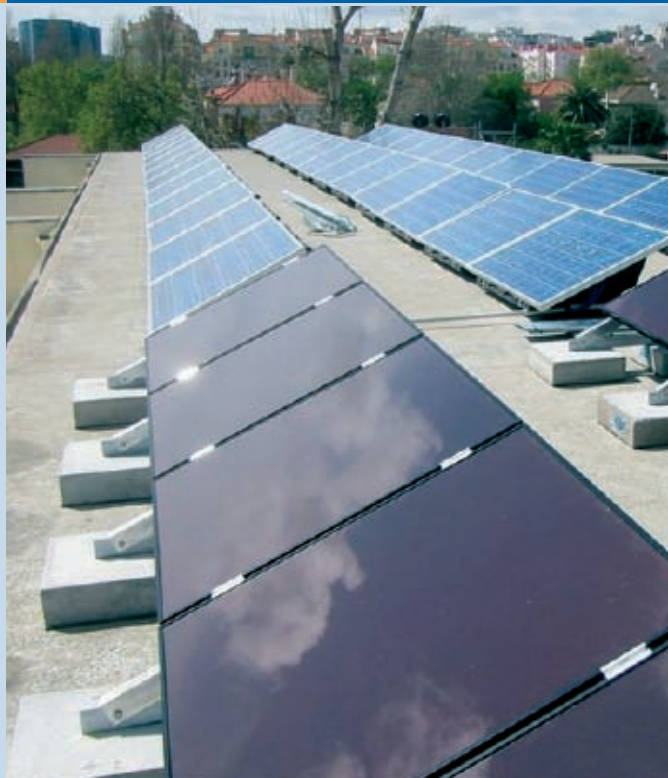
Fig. 2 - German School: 25 kWp grid-connected PV system at the Lisbon German School (photo courtesy of Jayme da Costa) .
