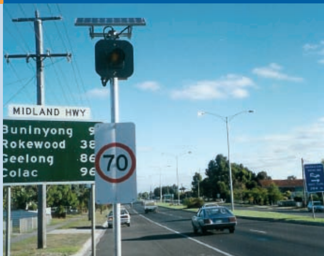
Fig. 4 - 50W system for a school crossing in Ballarat, Victoria (photo BCSE).
