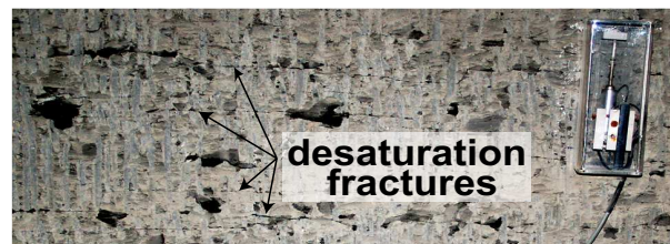
Figure 1.6: Horizontal desaturation fractures at the wall of the 1996 excavated gallery. On the right: measuring device for crack aperture.
