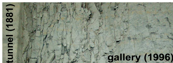
Figure 1.5: Fractured zone around the 1881 excavated tunnel. View of the floor of the 1996 excavated gallery.
