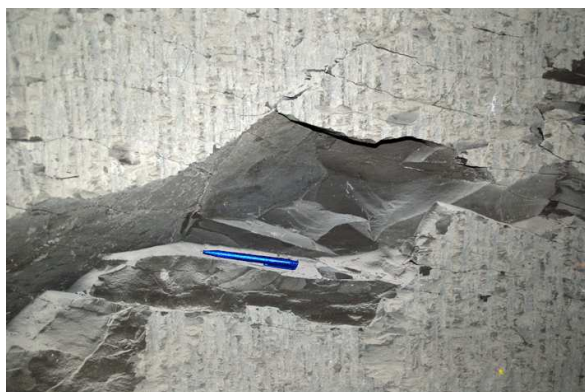
Figure 3.55: Spalling at the wall of the gallery. The darker area signifies the rock surface with higher water content, which has been exposed to the atmosphere quite recently.
