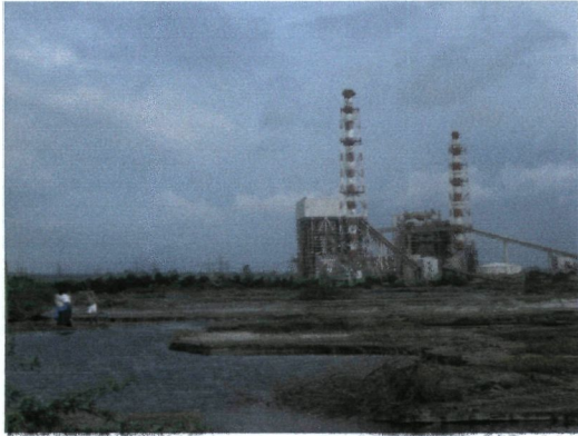
Ash pond area flooded with water
