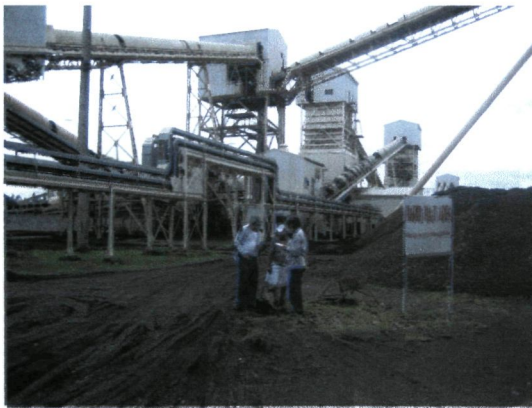
Near coal yard area
