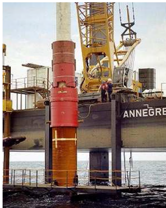
Figure 1: Hydraulic hammer on a pile of FINO1
