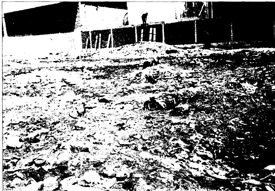
Plate (4): Streets inside the industrial area over crowded With old dumpings for liquid and solid wastes, which have Affected the walls of one of the factories.
