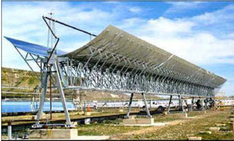
Figura 5. Colector de canal parabólico EuroTrough ([www.eurotrough.com](http://www.eurotrough.com))
