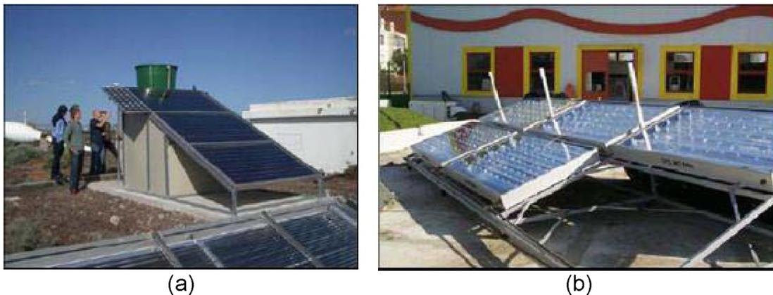
Figura 22. (a) Colector plano del Fraunhofer Institute for Solar Energy Systems. (b) CPCs de la empresa portuguesa Ao Sol.
