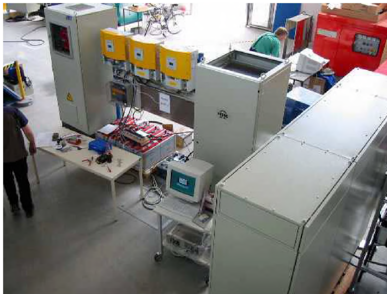
Figure 10: Electrical system testing at ISET.
