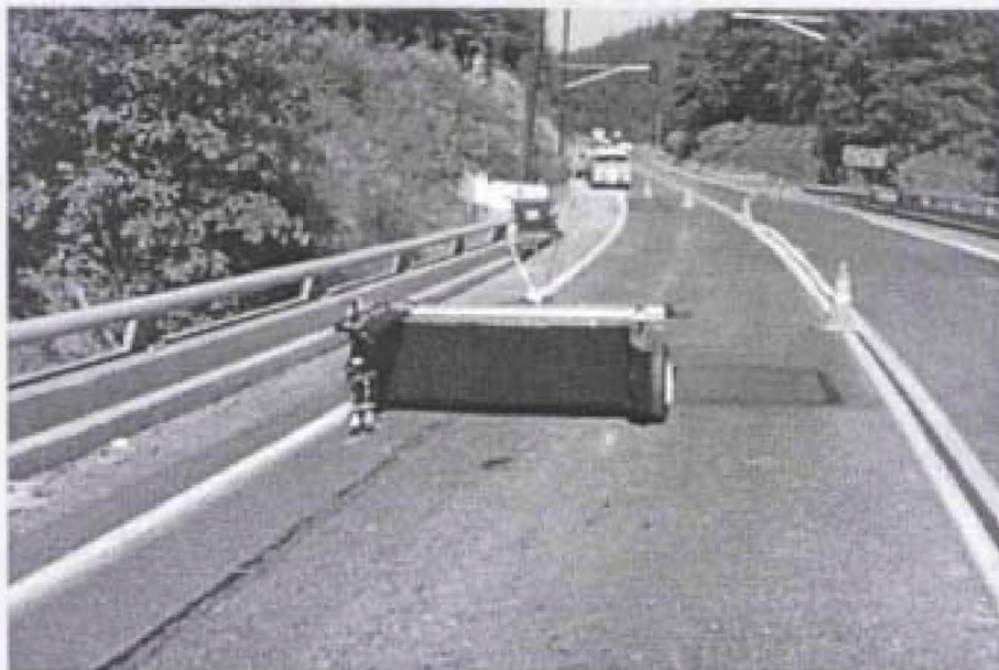
PERES surveying a bridge deck.
