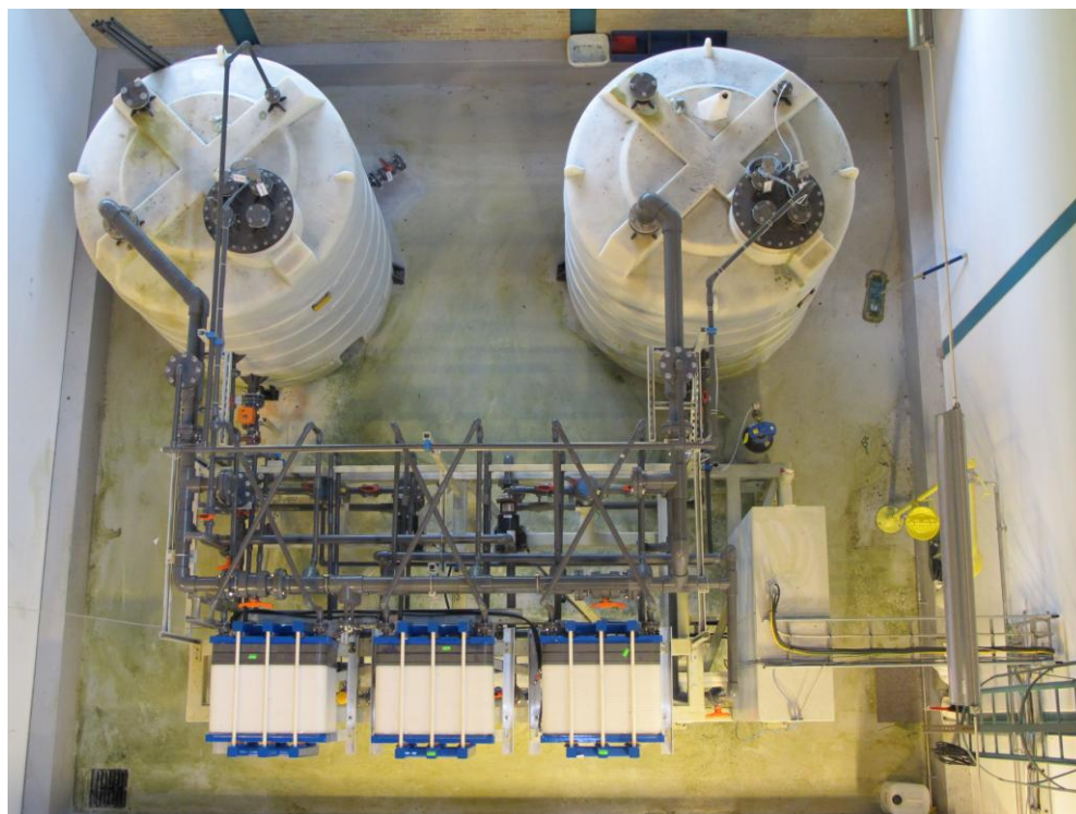
Figure 4 Vanadium battery installation seen from above: electrolyte tanks in the back, 3 cell stacks at the front.
