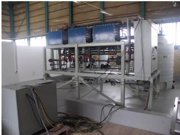
Figure 3: Photograph of the vanadium battery at SYSLAB during installation. To the right, the system components are listed.
