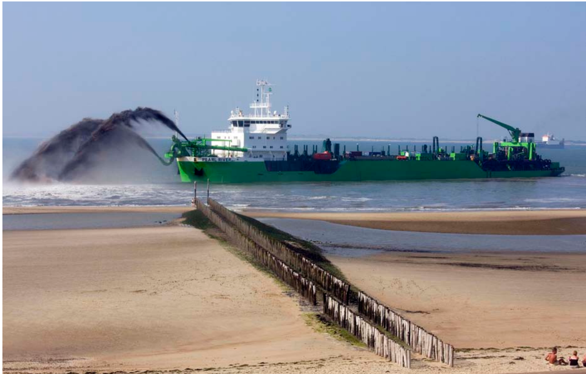
Figure 4.2: Rainbow method for transferring nourishment material ashore
