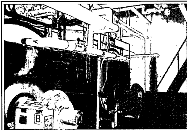
This large complex in the Bronx with 361 units now has a pair of new energy-efficient 200 horsepower boilers and a newly designed distribution control system.
